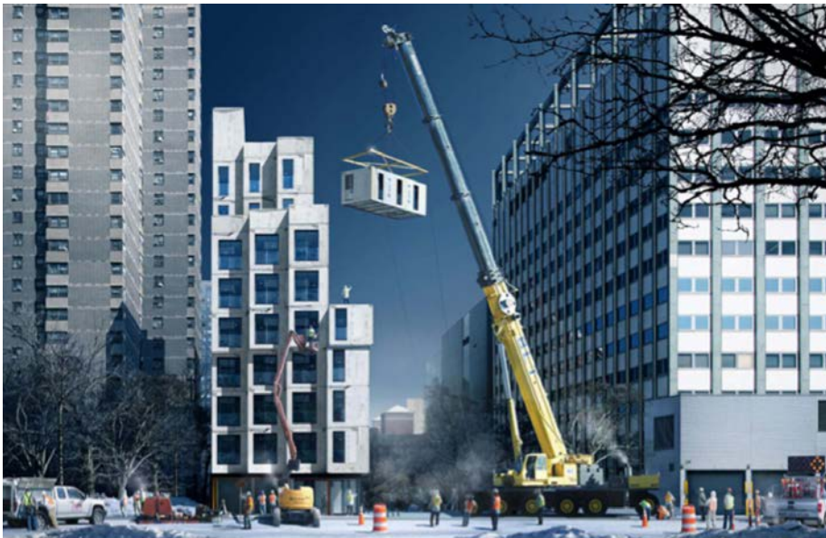
Rendering of installation of modules at My Micro New York pilot project site. Source and image credit: nArchitects.
