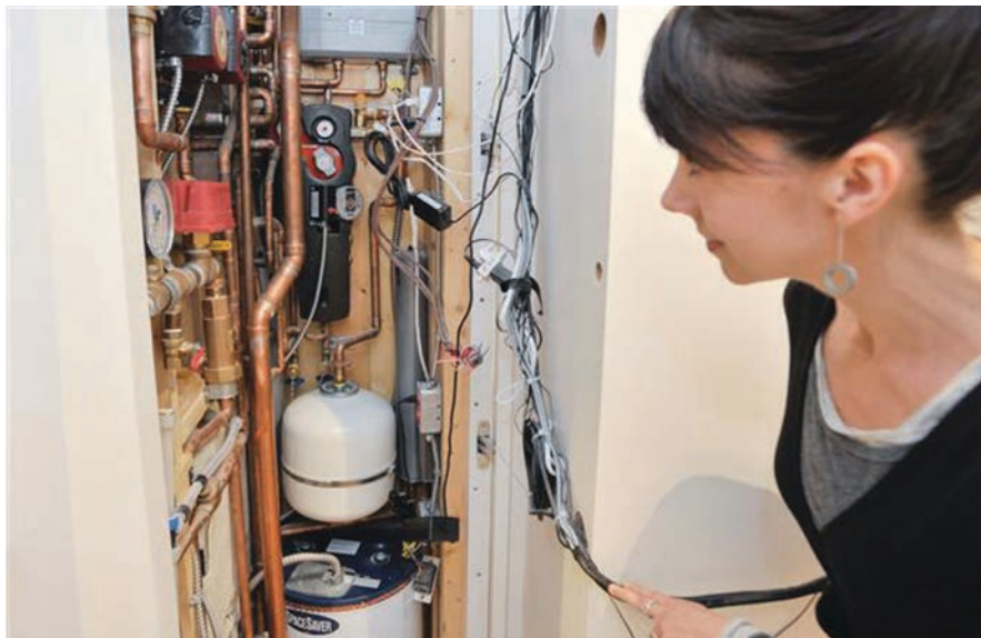
A glimpse at the solar thermal capillary heating and cooling system in the L41 micro home by Michael Katz and Janet Corne. Photo Credit: Jason Payne, Vancouver Sun.
