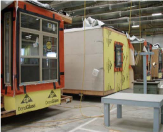
Factory-built construction of Modular Units for Panoramic Interests micro-apartment project in San Francisco by Zeta Communities. Source and image file: Panoramic Interests and Zeta Communities.
