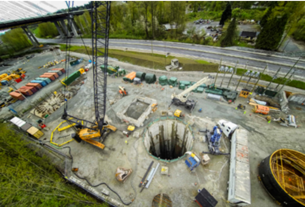
COVER: Construction of a vertical shaft at the Port Mann water tunnel. See article on page 38. Photo by Metro Vancouver.
