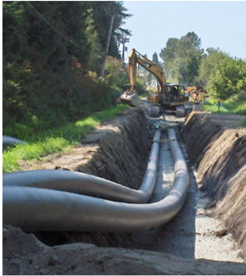
Sanitary force main construction in Campbell Heights (above and near right) and at Port Kells pump station (far right).
