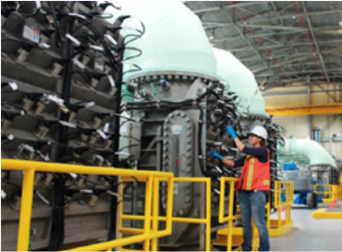
Coquitlam Water Treatment Plant UV reactors (above); installation of a three-metre-diameter Metro Vancouver sewer in Surrey to service growth in the city and township of Langley, and in Surrey (right).
