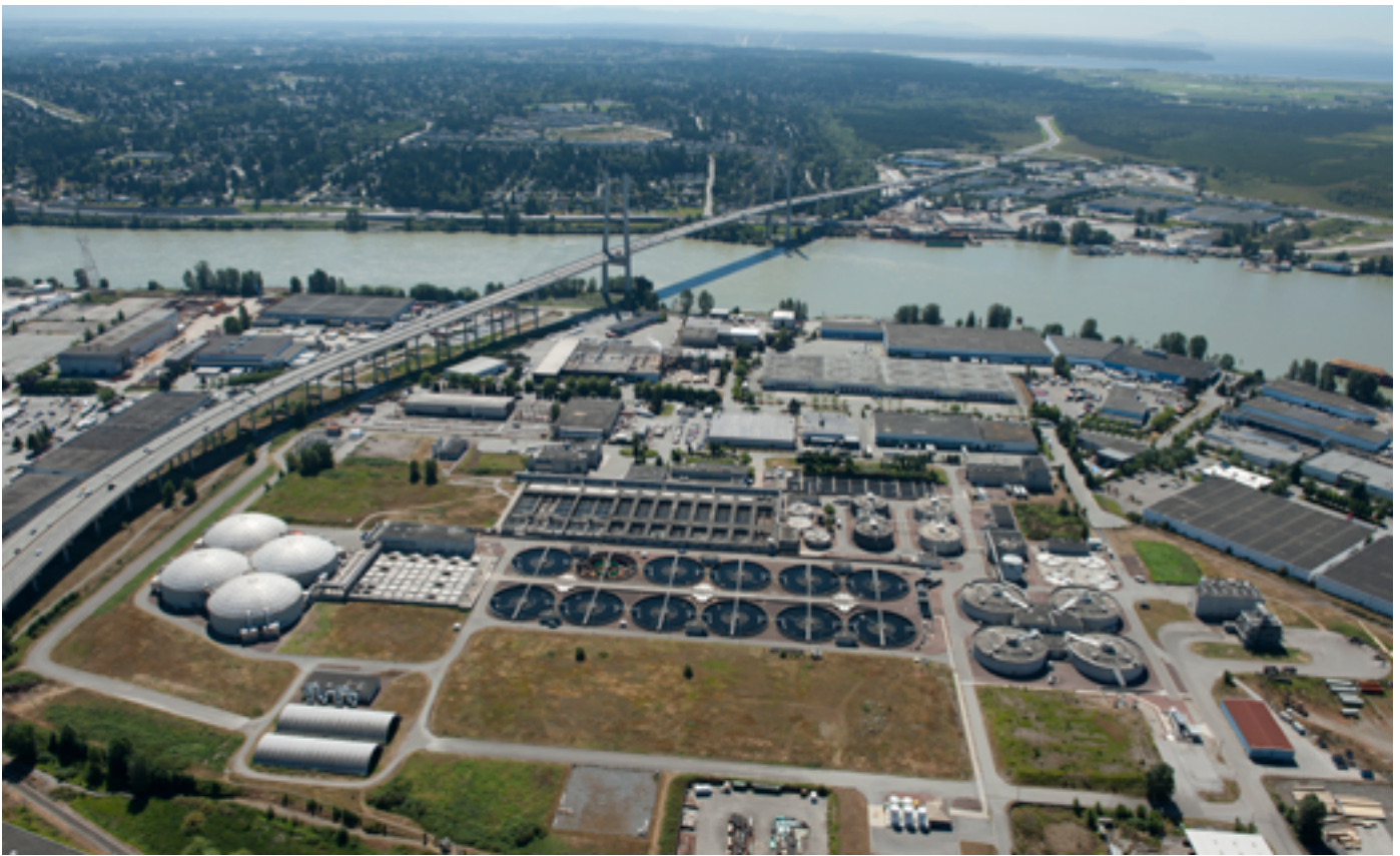
Annacis Island Wastewater Treatment Plant (above); cogeneration engines at Iona Island Wastewater Treatment Plant (next page, above); analyst at work with a Metrohm instrument, which automatically analyzes pH, alkalinity, and conductivity of liquid samples (next page, below).
