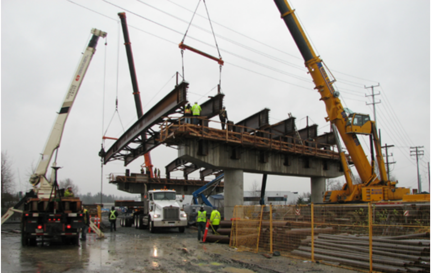
Construction of a new rail overpass.
