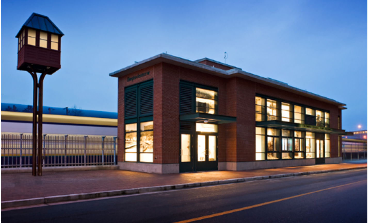
Columbia Pump Station is designed to integrate with Vancouver's historic Gastown neighbourhood.
