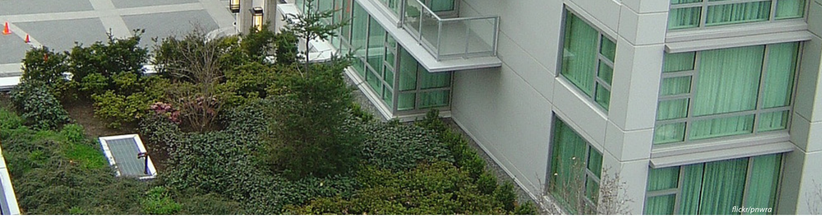
Green roof at the Marriott Hotel in Victoria.
