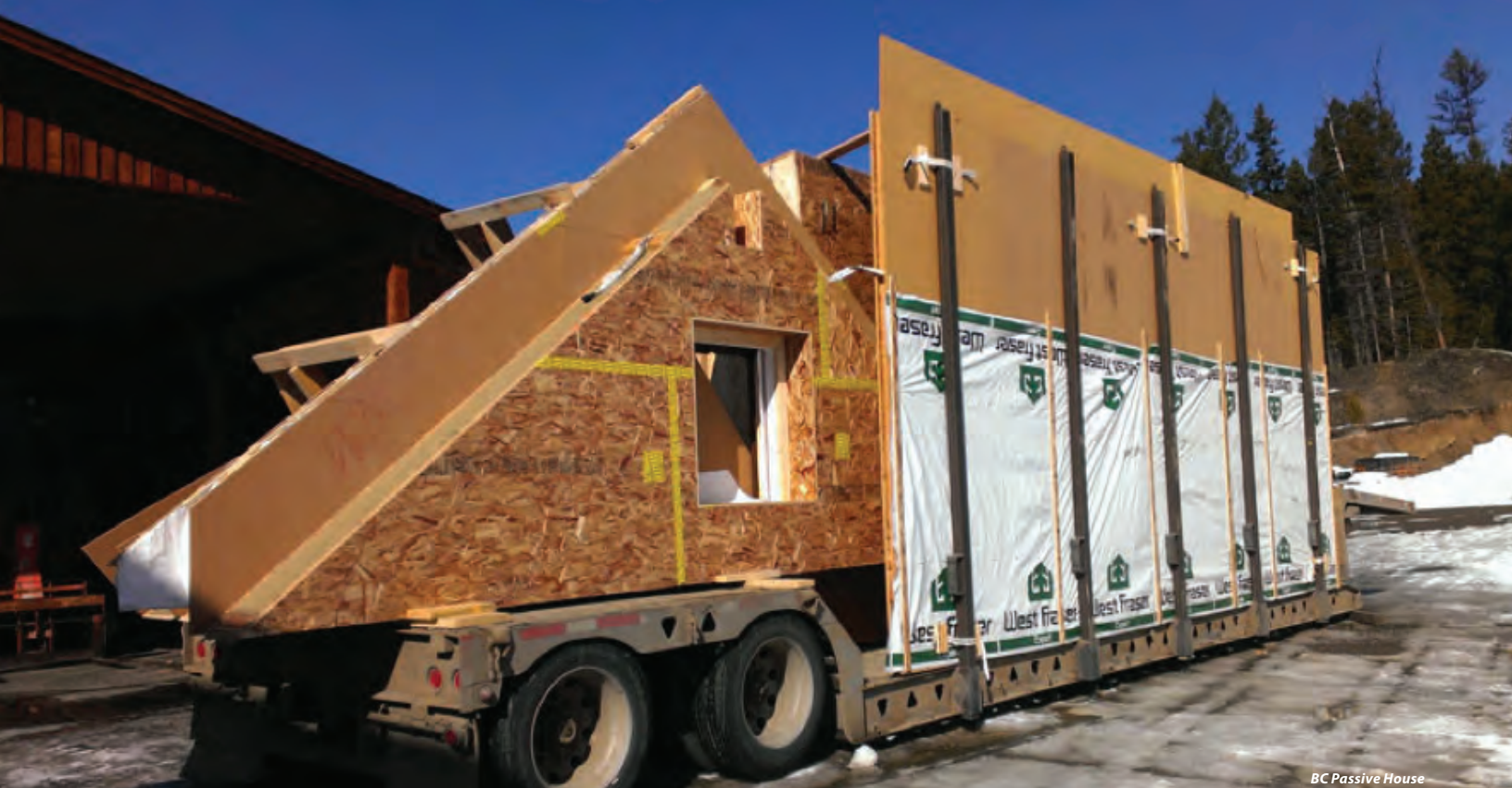
Truck delivery of Fort St. John's passive house, including modular roofing.
