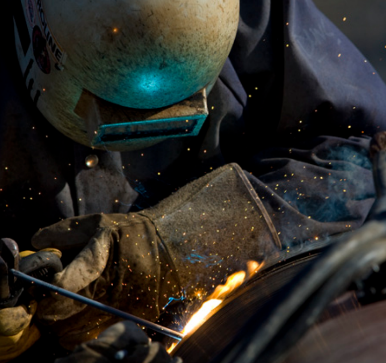
A worker welds two sections of pipe together on Enbridge's Waupisoo pipeline in Northern Alberta (2007). Photos and map provided by Enbridge.
