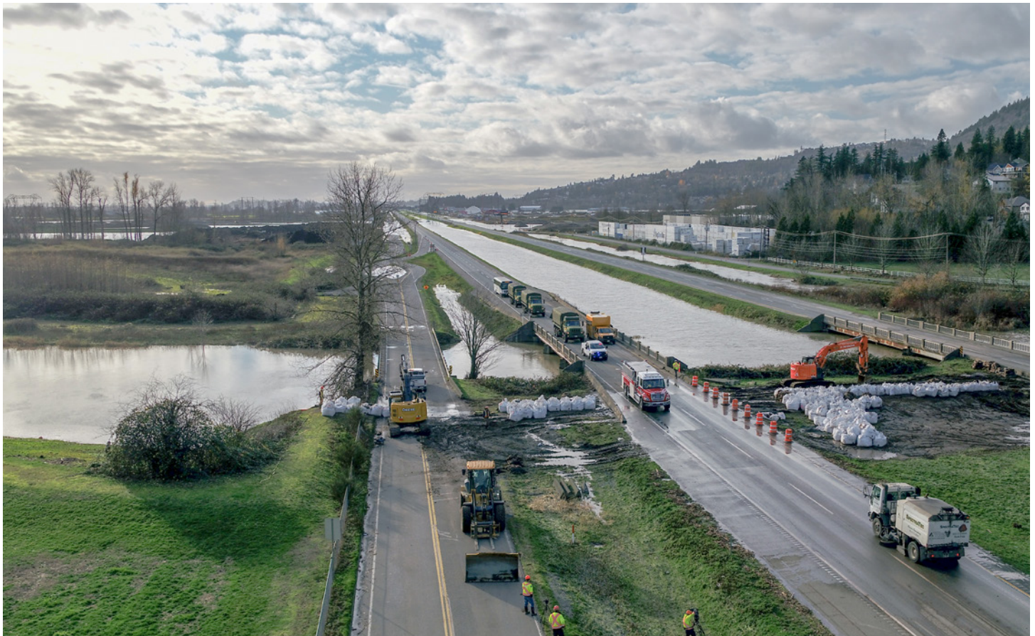
Top: Tiger dams were set up on Highway 1 in Abbotsford to hold back Sumas River flood waters, November 28, 2021. Above: Military traffic rolling out on BC Highway 1 after the removal of the temporary tiger dam across the highway in Abbotsford, December 2, 2021. flickr/BC Ministry of Transportation and Infrastructure
