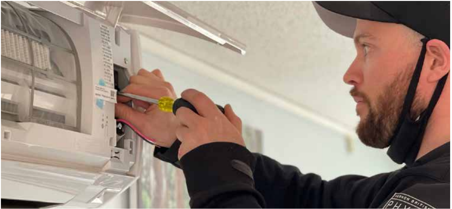
Ductless mini split AC installation. flickr/Phyxter Home Services (Phyxter.ai)
